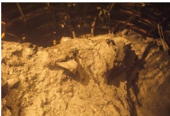
Photograph 4 Close – up view of 5.5m thick gougy shear zone with flowing condition tackled with fore-polling and multiple drift que.
