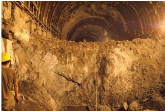
Photograph 5 Benching through gougy shear zone.
